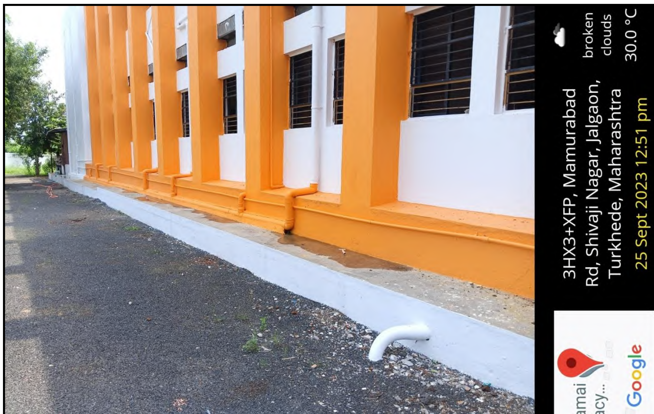
Geotag Image: Borewell Recharge by Rainwater pipeline
