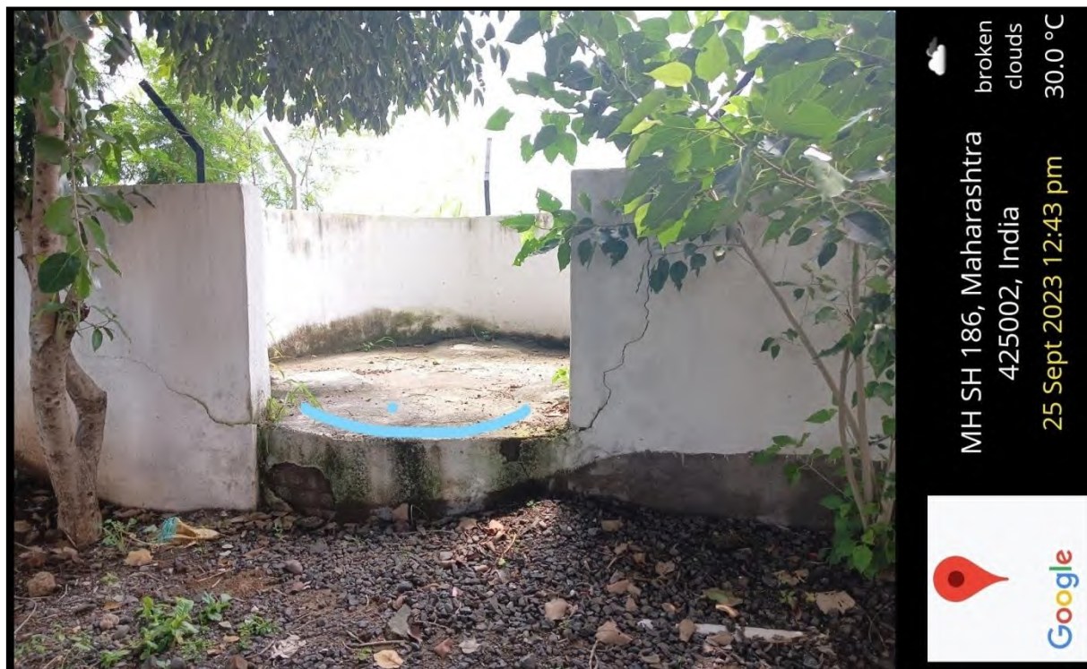
Toilet West Tank
