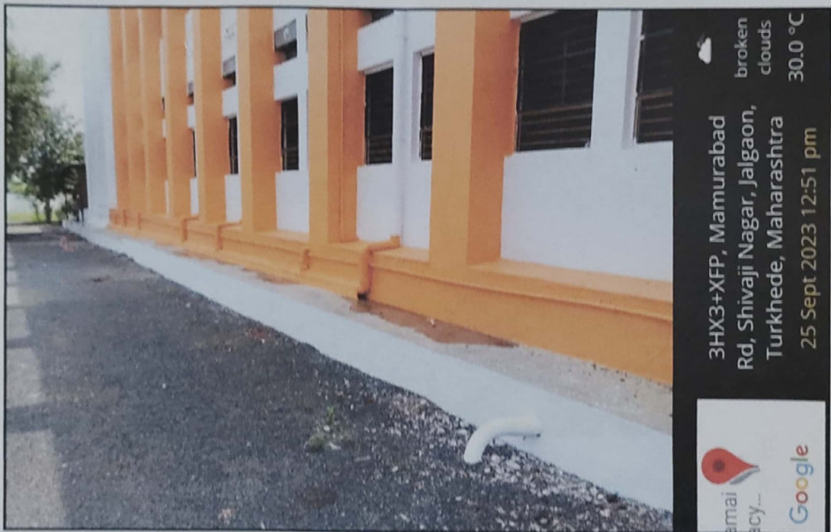
Geotag Image: Borewell Recharge by Rainwater pipeline
