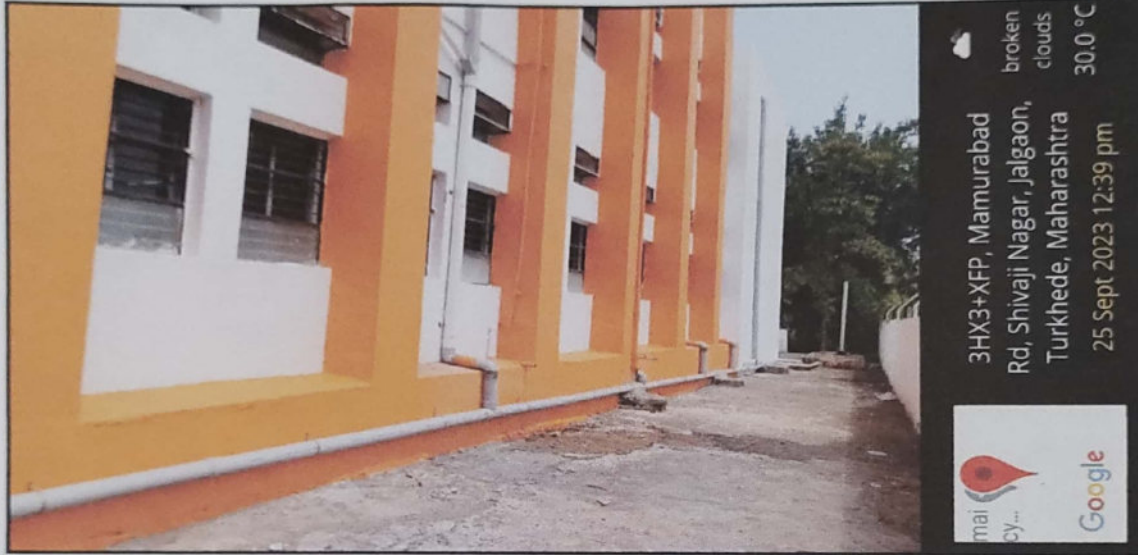
Geotag Image: Groundwater Recharge by Rainwater pipeline
