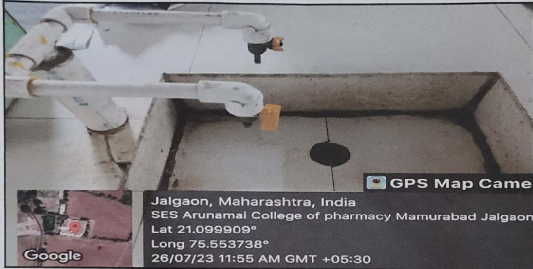
Geotag Image: Water-saving low-flow faucets
